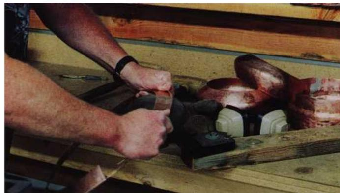
Figure 10. Once the rim has its edge rolled, it is hand-formed to a circular shape. The two ends are soldered together and it is ready to be attached to the battens and cap.
